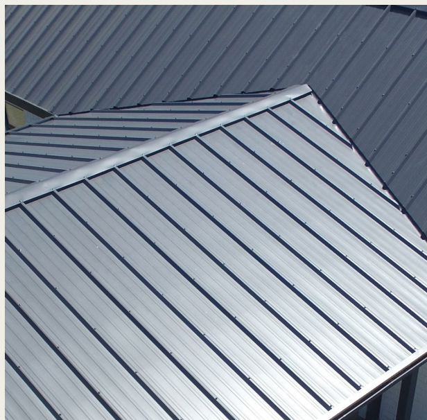
Solar Rib Roofing
