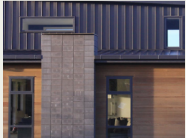
Stack bond masonry block
