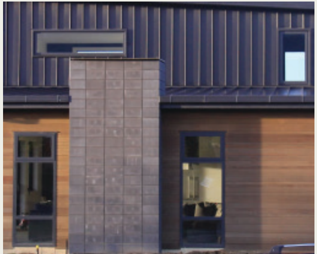
Stack bond masonry block
