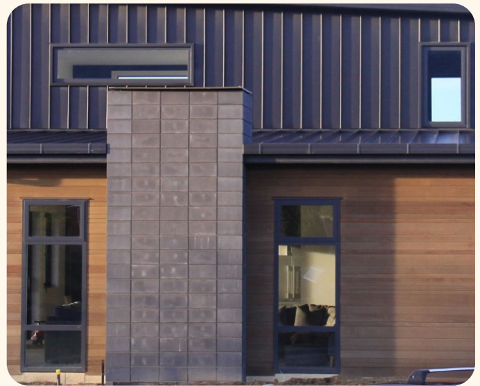
Stack bond masonry block
