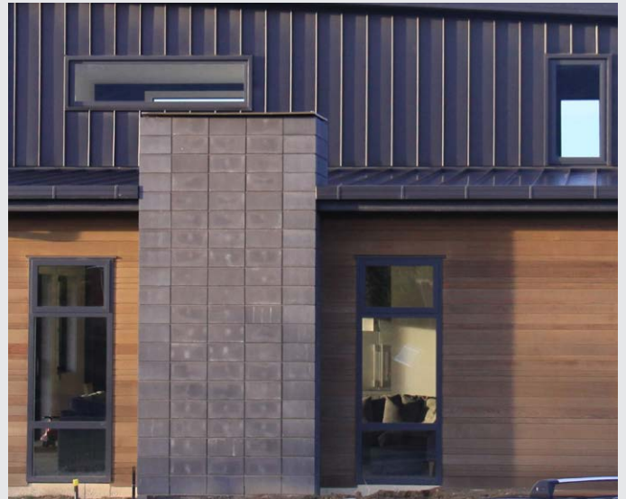
Stack bond masonry block
